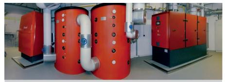
The most advanced technology in-situ at the Mercedes-Benz commercial vehicle centre in Frankfurt: centralised heating system with a PowerBloc CHP plant, an UltraGas<sup>®</sup> gas condensing boiler, buffer storage tanks and other system components
